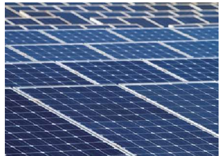
Solar Array Load Testing
